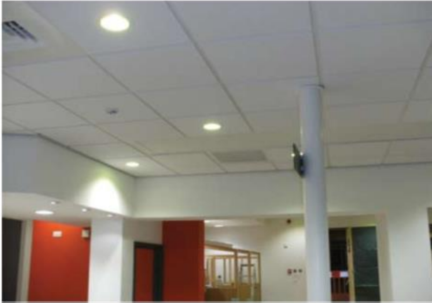
Flintshire County Council
